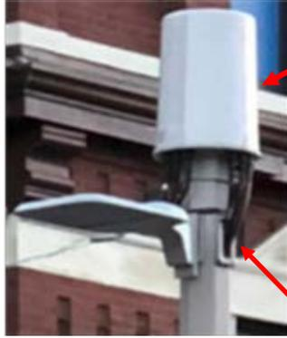
Conduit, mounting bracket, and other hardware must be hidden from view
