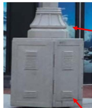
Cantenna must include a smooth transition between upper pole and Cantenna attachment
