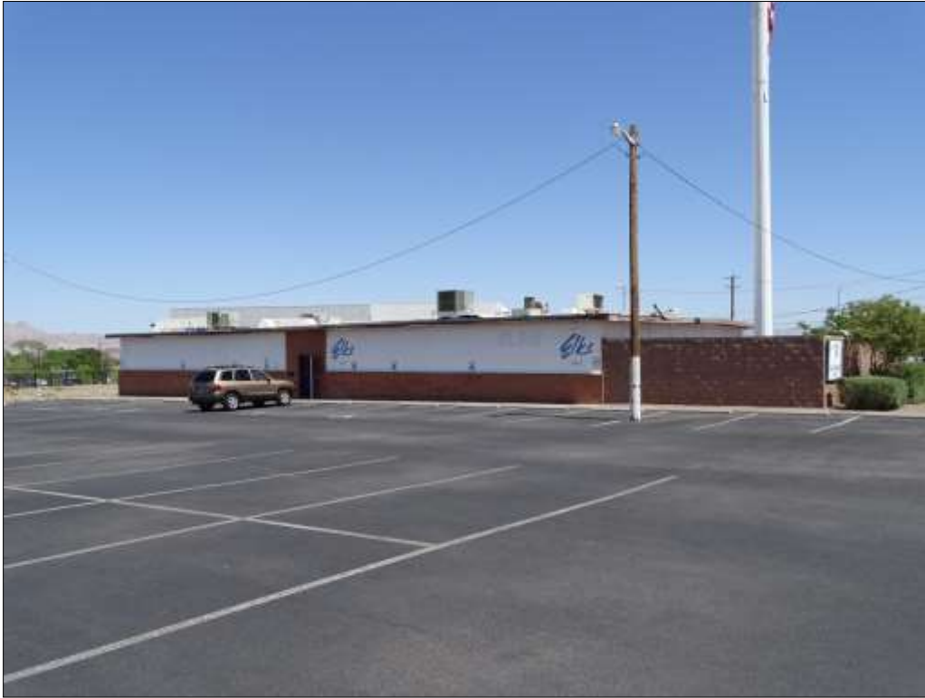
Photograph 48. The Elks Lodge as it appears today, facing northwest (North Wind, 2016).
