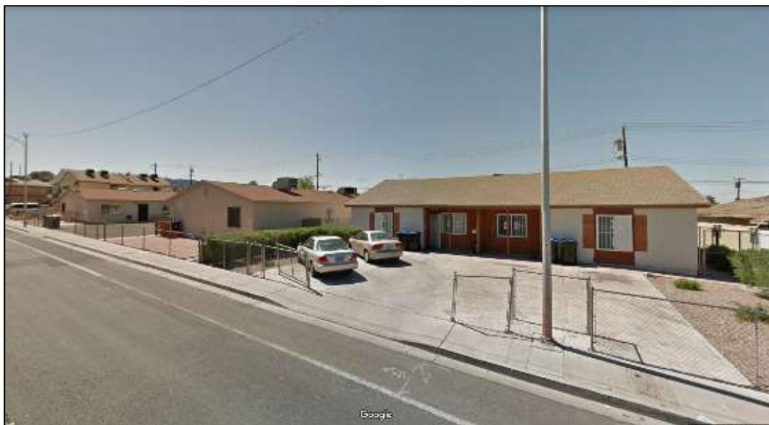
Photograph 34. Multi-family dwellings along North Major Avenue in Bulloch Subdivision No. 1, facing southwest (Google Earth, 2016).
