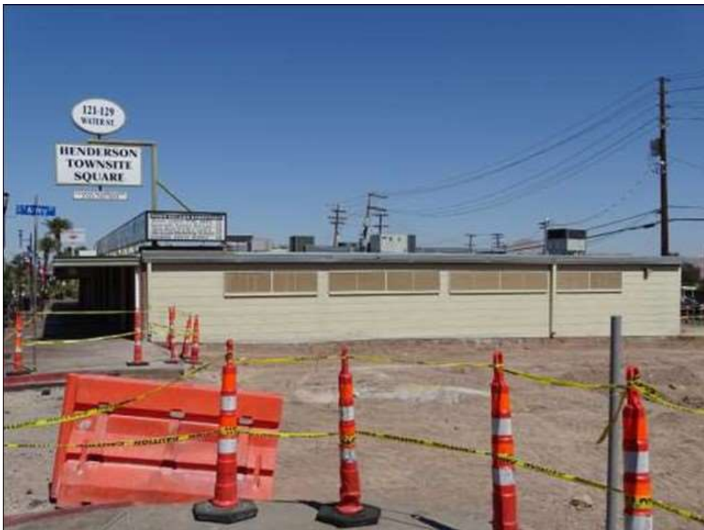
Photograph 36. Example of a commercial building at 121–129 Water Street, facing south (North Wind, 2016).
