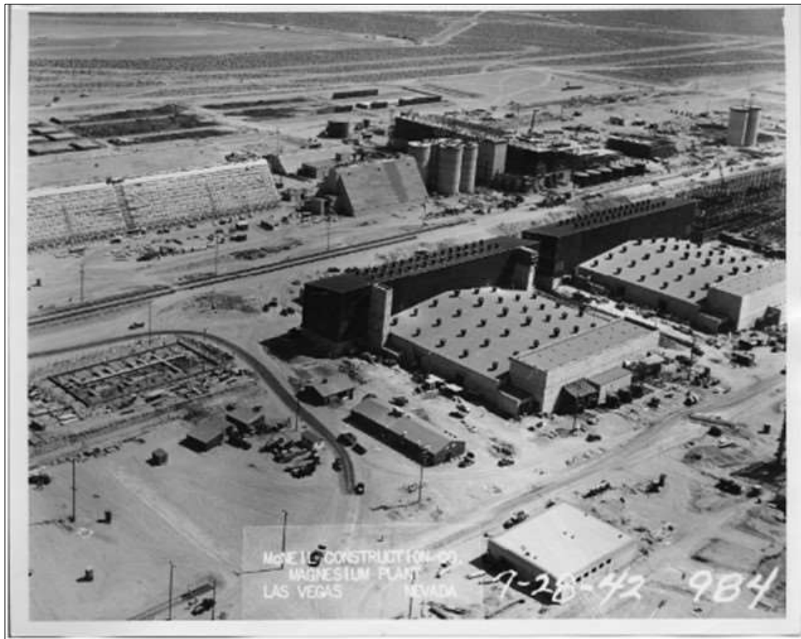
Photograph 23. Aerial view of BMI plant buildings, July 1942 (Image courtesy of Henderson Public Libraries).
