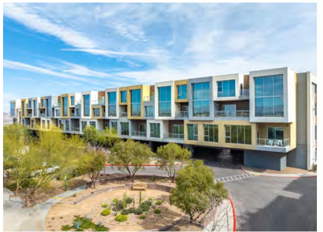
Multifamily with parking integrated under the building.
