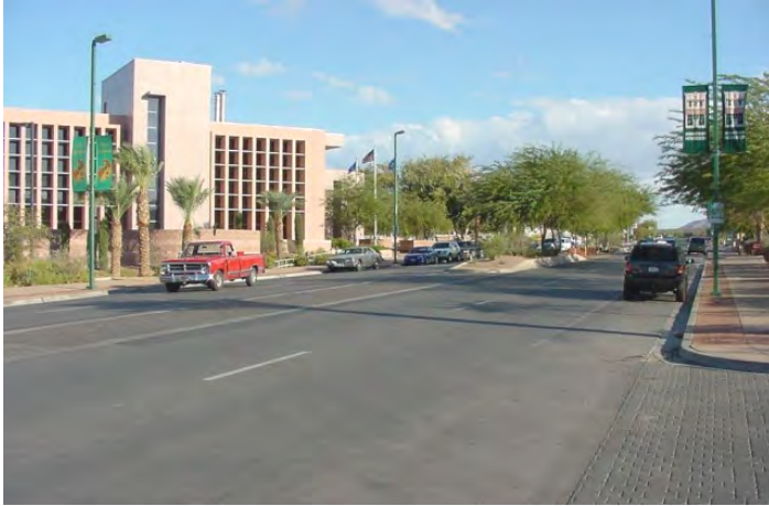
Figure 16—Justice Center—East side: Recent construction, no pedestrian orientation towards Water Street.
