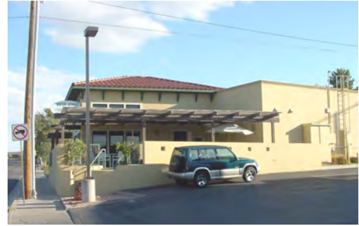
Figure 38—Coffee shop on Water Street.
