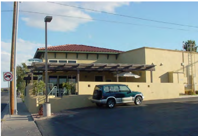
Figure 20—Water Street Coffee Company—West side: Strong street presence, inviting outdoor seating.
