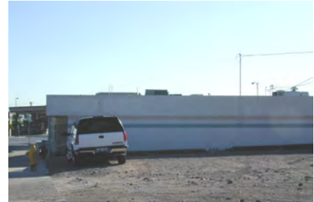
Figure 37—Code requirements dictated that the business sign that had been painted on this wall had to be removed.
