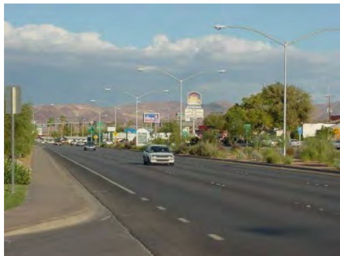
Figure 3—Lake Mead Drive Northwest of Downtown.
