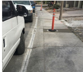
Saw-cutting material should not run down the street. BMPs should be in place at the source to prevent this.
