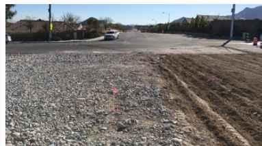
Stabilize construction site entrances/exits to minimize track out of dirt and mud. Entrances/exits should funnel traffic so vehicles use track out BMPs.
