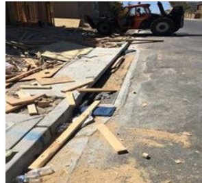
Pollutants such as sawdust and sediment should be swept from the curb and gutters.
