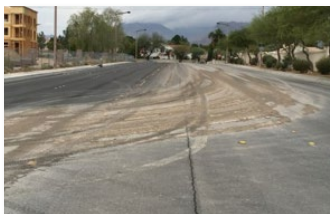
Stabilize construction site entrances/exits to minimize track out of dirt and mud. Entrances/exits should funnel traffic so vehicles use track out BMPs.
