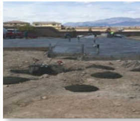
Concrete washout/waste should not be placed on the ground. It should be placed in a leak-proof container.
