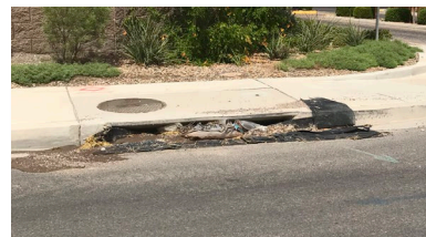
BMPs should not be ripped, falling into the drop inlet or placed on or next to the grate in publicly traveled areas. BMPs should be maintained, sediment and trash should be removed.
