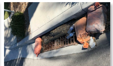
BMPs should not be ripped, falling into the drop inlet or placed on or next to the grate in publicly traveled areas. BMPs should be maintained, sediment and trash should be removed.
