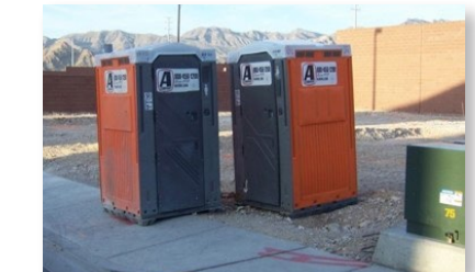
Toilets could tip and spill into the street. Portable toilets should be secured and behind curb.
