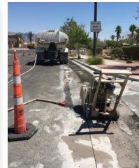
Saw-cutting material should not run down the street. BMPs should be in place at the source to prevent this.
