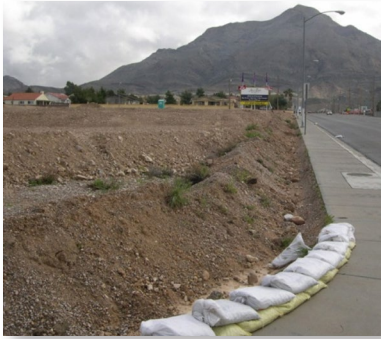
Wattle is secured, and the property has back-of-curb cutbacks.
