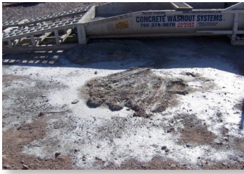
Concrete washout/waste should not be placed on the ground. It should be placed in a leak-proof container.
