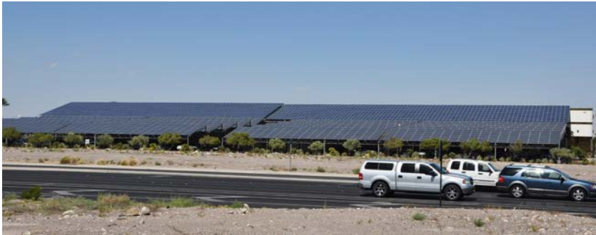
Solar canopy structures in parking lots provide a dual function of serving as a supplemental power source and providing additional shade.
